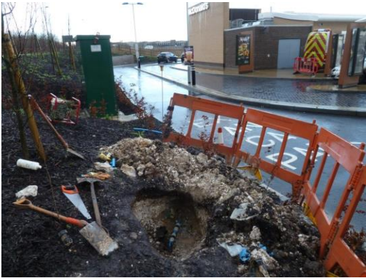
Location of repair
