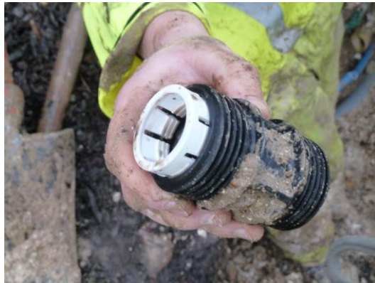
Incorrectly inserted gripper ring
