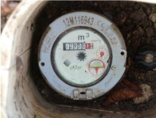
Water meter after repair
