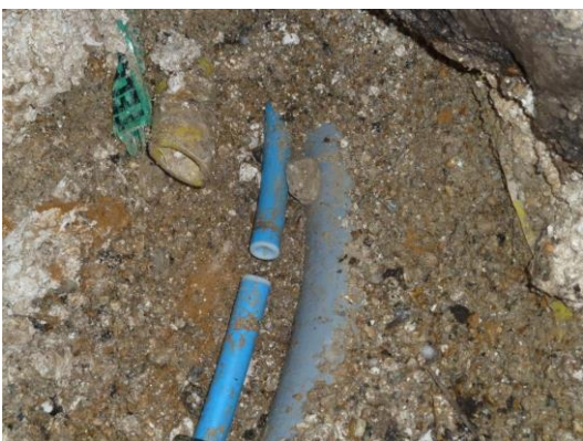
Pipe ends cut too short
