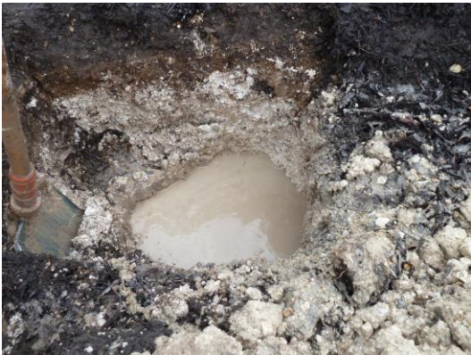
Water found under surface of ground
