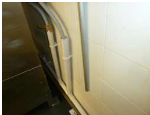
Waste pipework to rear of ice machine
