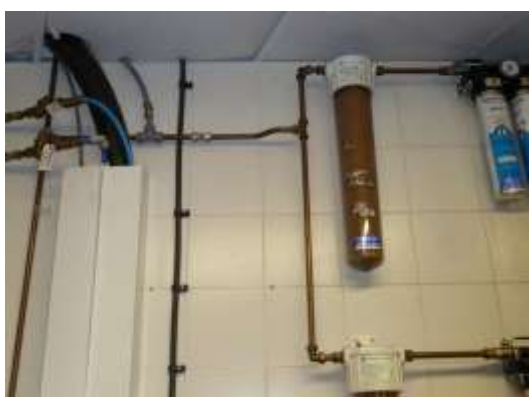
Cold water inlet pipework to ice machine
