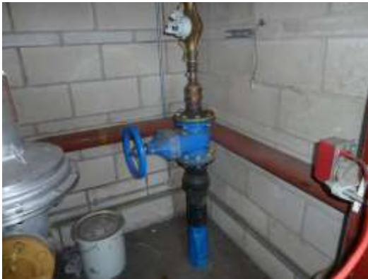
Meter location and rising main in plant room
