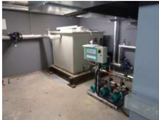
Water tank and pumps
