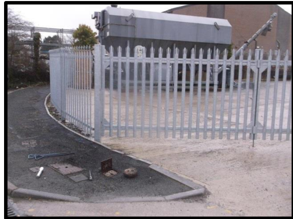
Picture 2 – Plymouth Water Meter Location
