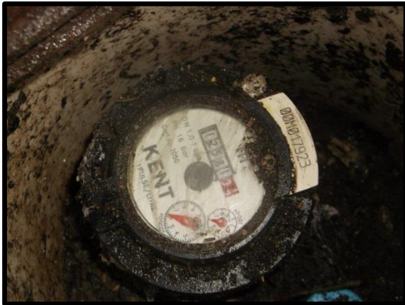
Picture 1 - Plymouth Water Meter
