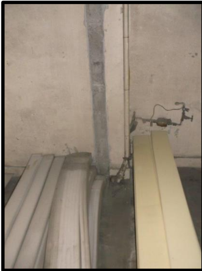
Picture 3 – Rising Main in the Warehouse
