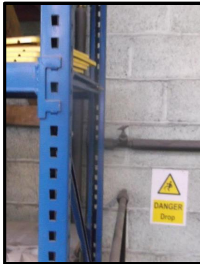
Picture 4 - Stop tap on left branch used to isolate the left branch supply
