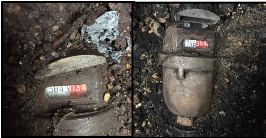
Picture 1 – Water Meter 076417 feeding the vacant offices
