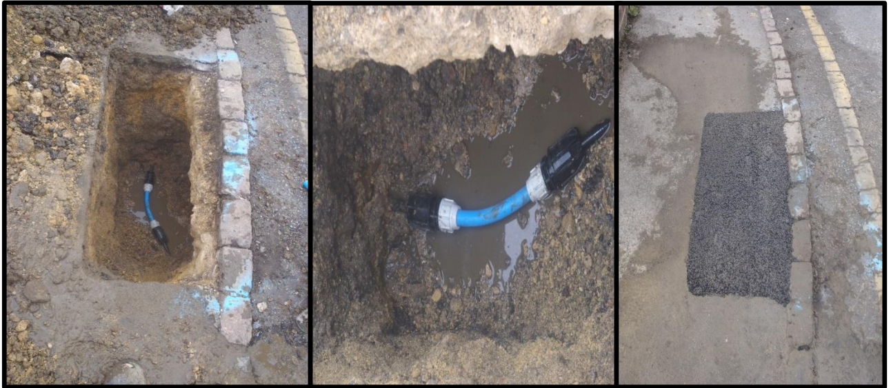
Picture 4 – The excavation in tarmac
