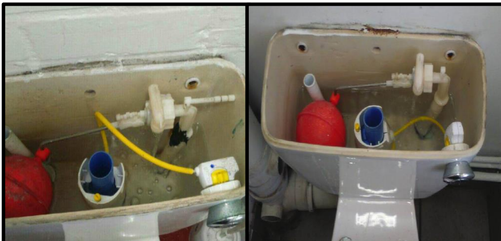
Both of the toilets upstairs were found to be constantly running due to broken ball valves within the toilet tanks
