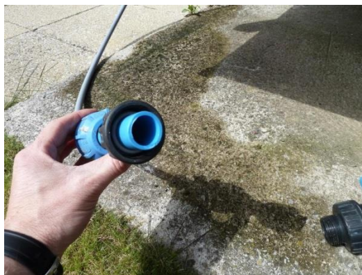
Insert missing from above ground pipework
