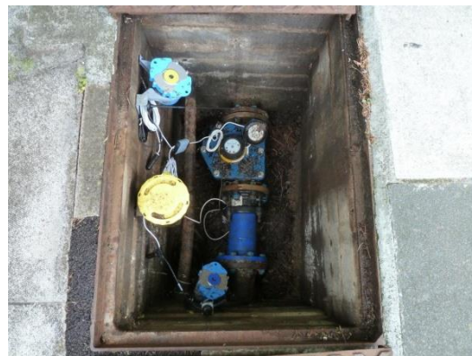
Meter chamber and loggers
