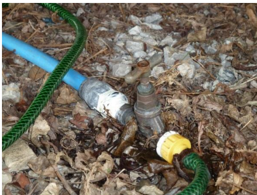
Leak on hose connection at Windsor plot 74
