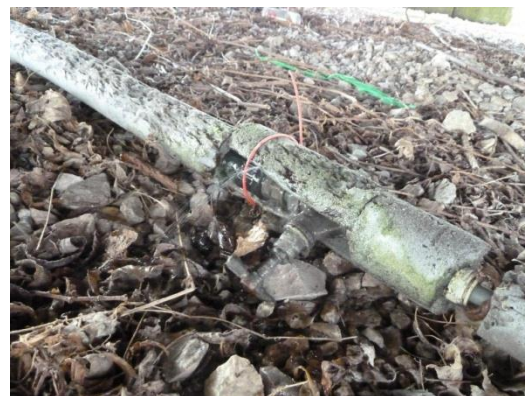
Leak on second stoptap to Windsor plot 74
