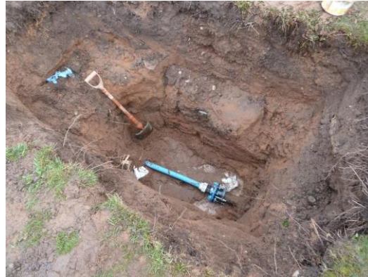
New connection in substation land
