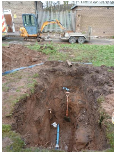
Line of main looking away from A52
