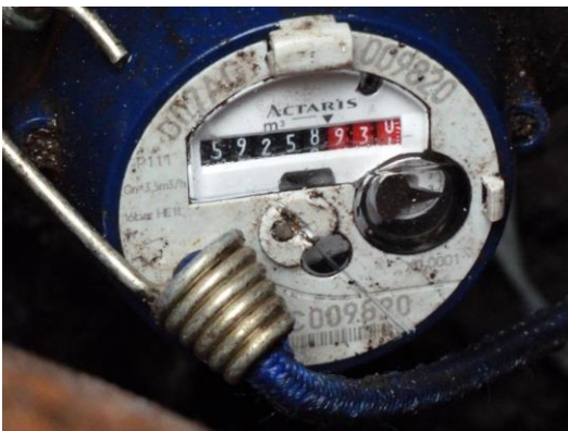
Water meter reading after repair
