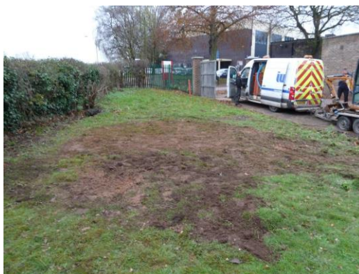
Reinstated excavation
