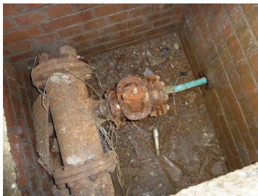
Section of sliplined pipework leading to workshops
