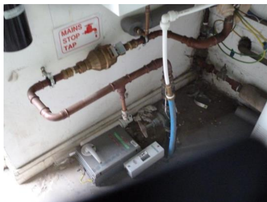
Meter location in plant room
