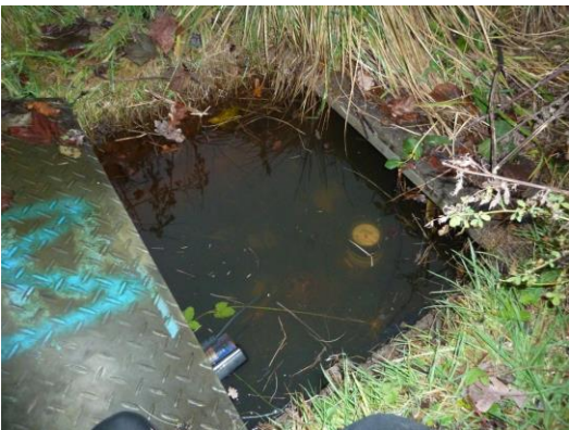
Main meter chamber (flooded)
