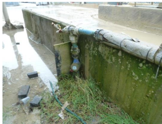
Meter location under mortar batching plant
