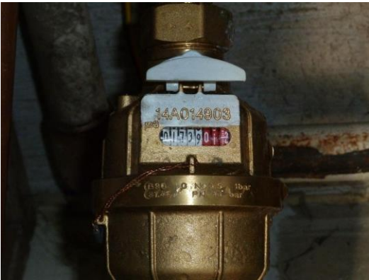
Unit A - Colas offices meter in gas meter cupboard
