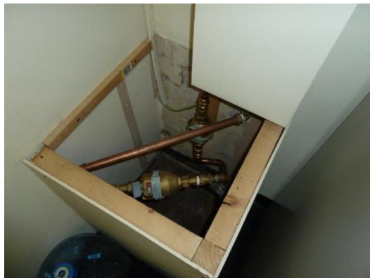
Unit C meter location
