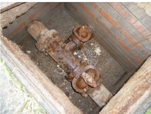
View of site pipework in chamber
