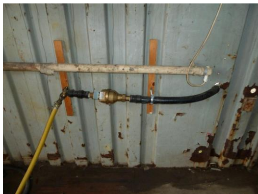
Compound X9 rising main in metal container
