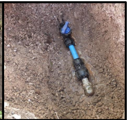
Picture 7 – Leak 2 repaired and stop tap replaced
