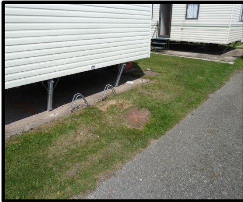
Picture 3 – Leak 1 location on stop tap at rear of plot HC8 (Valve under chamber lid)
