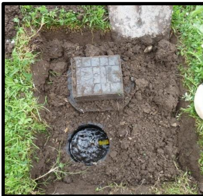
Picture 5 – Leak 2 location at rear of plot RA3 (Chamber lid was completely covered over with turf)
