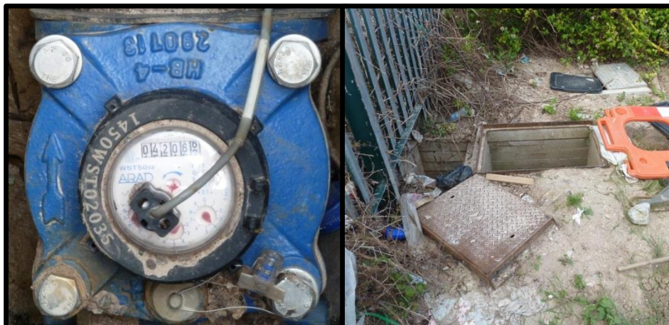
Picture 1 – Water meter 1450WST02035
