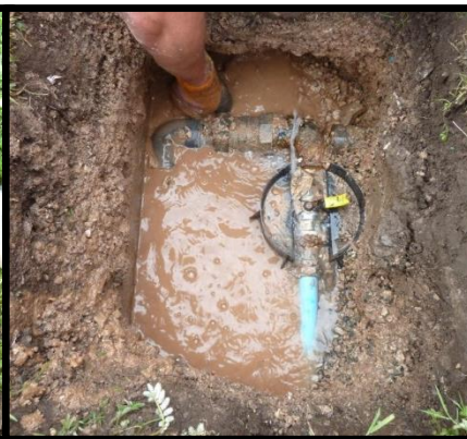
Picture 6 - Leak 2 excavated
