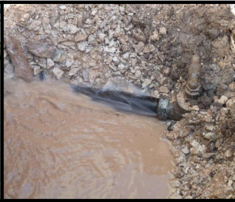
Picture 4 – Leak 1 uncovered found to be blown olive/compression nut on stop tap
