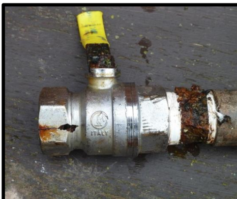
Picture 7 – Cause of Leak 2 was due to split in Valve
