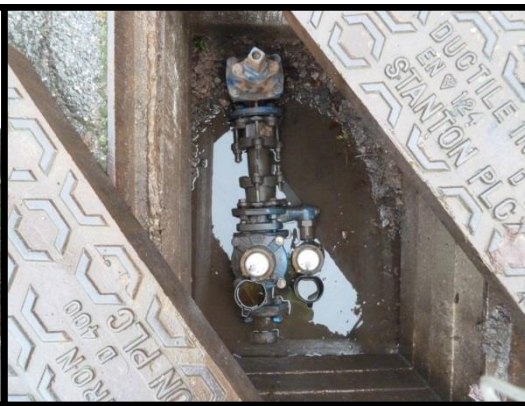
Picture 2 – Inside water meter chamber
