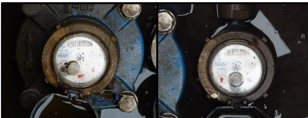
Picture 3 – Main Water Meter 0850Cm0015
