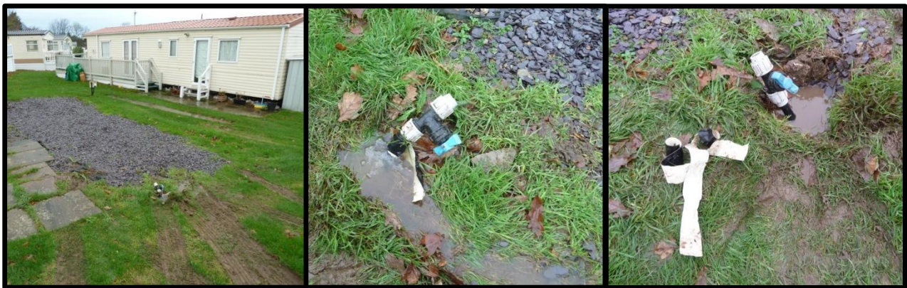
Picture 5 – Location of leak – Plot T11
