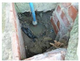
Leak location 4 - leak on riser to 9 Hillview
