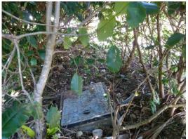
Valve chamber located under bushes – needs to be made more accessible
