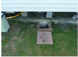
Leak location 3 - leak on riser to 8 Hillview
