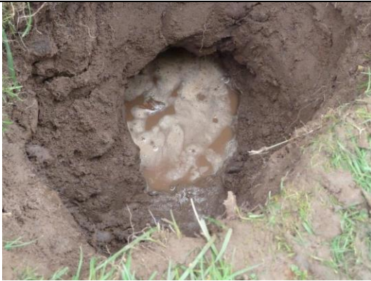
Trial excavation to pinpoint leak by 35 Morton Mews
