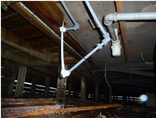
Leak coming from floor underneath mobile home
