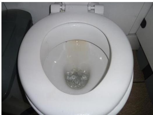
Overflowing WC cistern in ladies toilets
