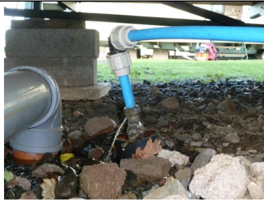
Leak on brass stoptap – plot 186 Bambi Court
