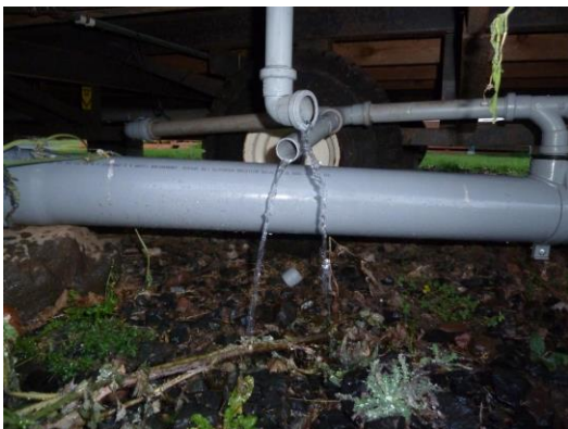
2x taps left on inside plot 445 Wool Park for frost prevention?
