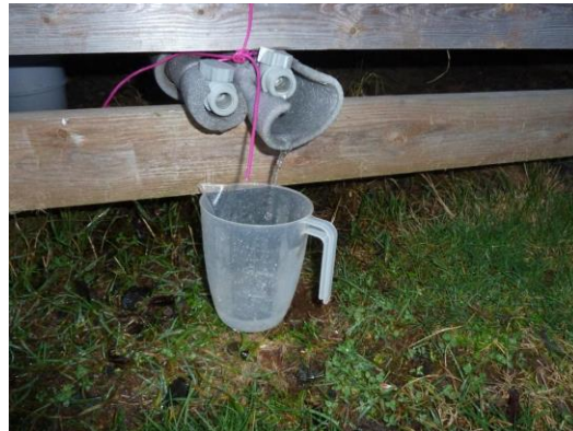
Measuring leak at plot 428 Wool Park
