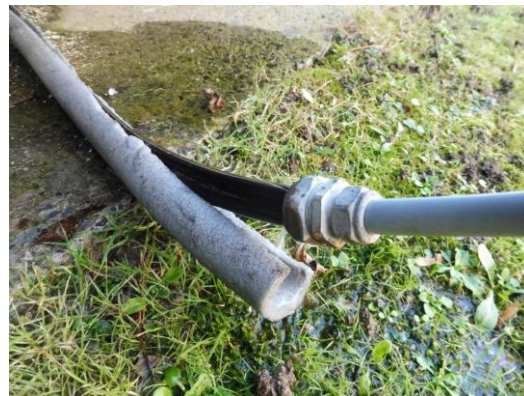
Leak on fitting Pembroke 25
