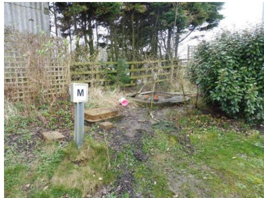
Main meter location
