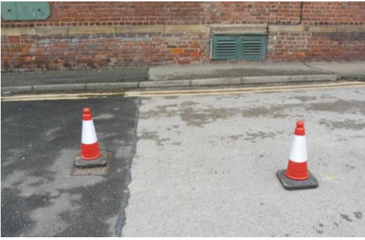
Valve (L/H cone) and service duct (R/H cone). Likely excavation point is between the two, taking care to avoid disturbing the service duct beneath
