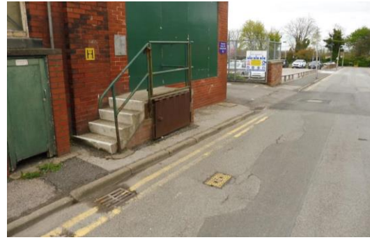
Hydrant leak on Barn Drive near Motor Road
