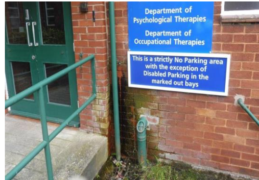
Overflow leaking from the Silver Centre
