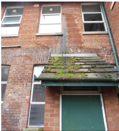
Overflow leaking rear of Health Clinic
