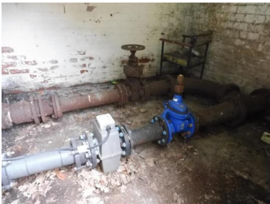
Meter location in room off Main Road
