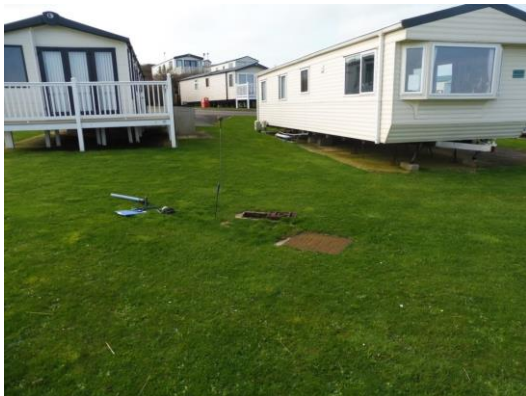
Location of leak on isolation valve between 5/6 Brampton Hedge
