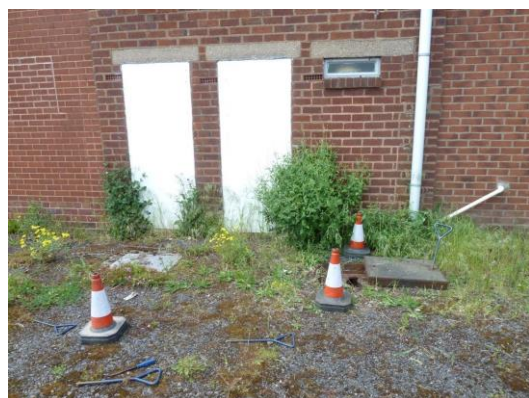
Line of main into building (cones marking route)
