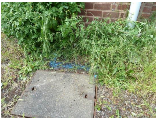
South Staffs area for investigation - IGNORE! Leak noise heard on building wall at this point believed to be originating from rising main
