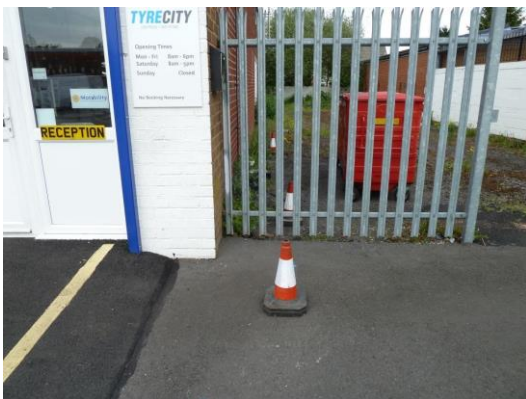
Likely leak position just in front of the metal fence (no surface noise to confirm correlation however)
