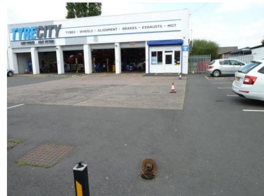
External line of pipework up to building (cones)
