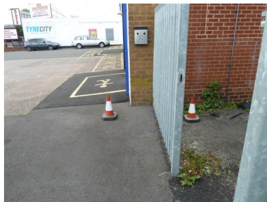
Excavate behind fence first (cone on RIGHT) to check leak isn't here before breaking into new tarmac in front of fence (cone on LEFT)
