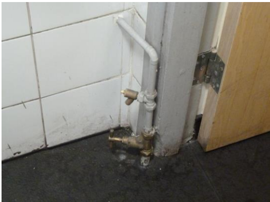
Rising main in staff WC
