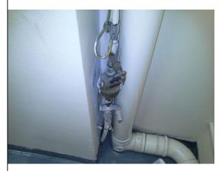
The External Water Meter on the footpath by the property boundary. The meter is moving. With the Internal supply isolated. The water loss was calculated to be 160 litres per hour, 3840 litres per day, this meter is not charged to the client account
