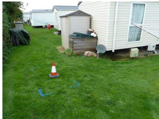
Leak location 2 – leak rear of 31 Thames Bank
