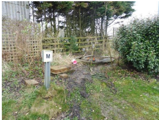
Main meter location
