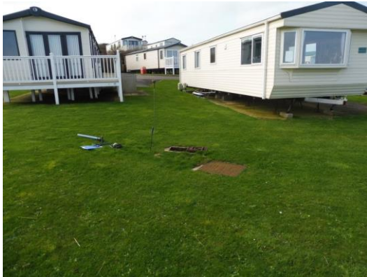
Location of leak on isolation valve between 5/6 Brampton Heights
